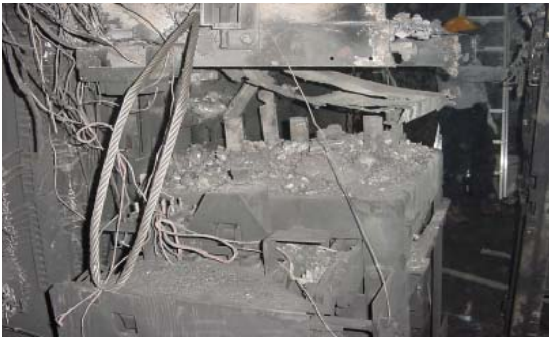
Damaged Breaker #17
